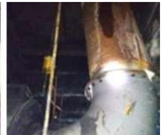
poor sealing
